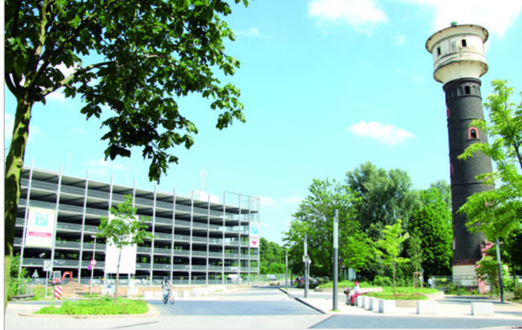
Parking garage by Konrad-Zuse-Platz
